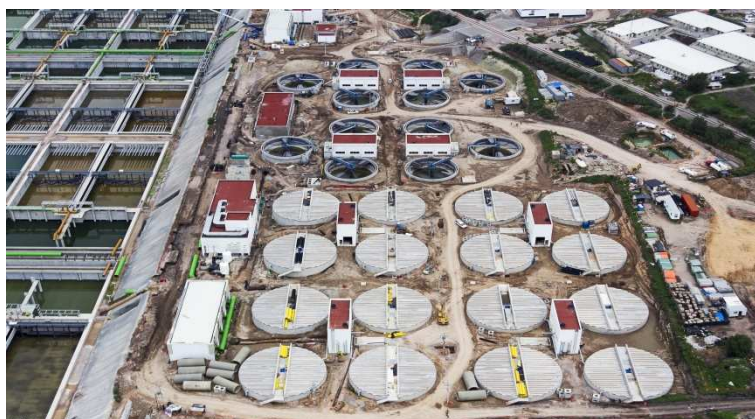
← Sludge Thickener Tanks
